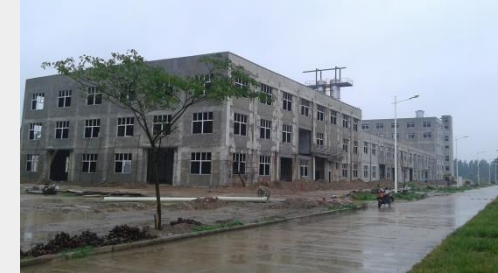
April 2015 – Workshop completed
