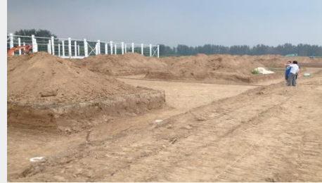
Aug 2014 – Workshop construction started
