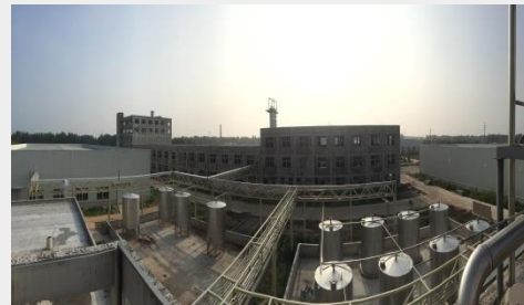
Oct 2015- Installation of facilities in workshop complete
