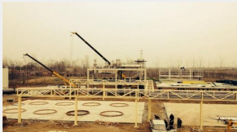
May 2015 – Installation of supporting facilities
